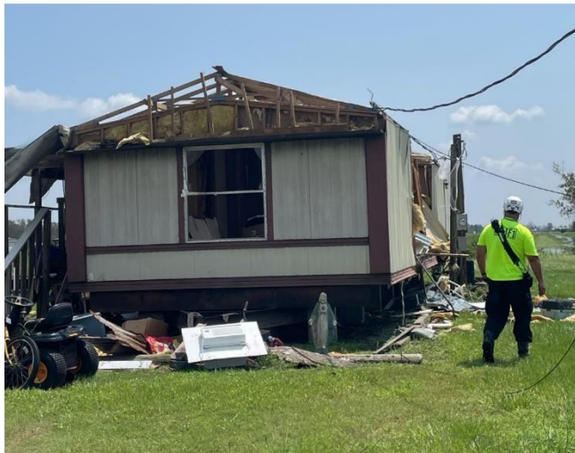
MI-TF1 search team member surveys a heavily damaged structure in St. James Parish, LA during the team's Hurricane Ida deployment.
