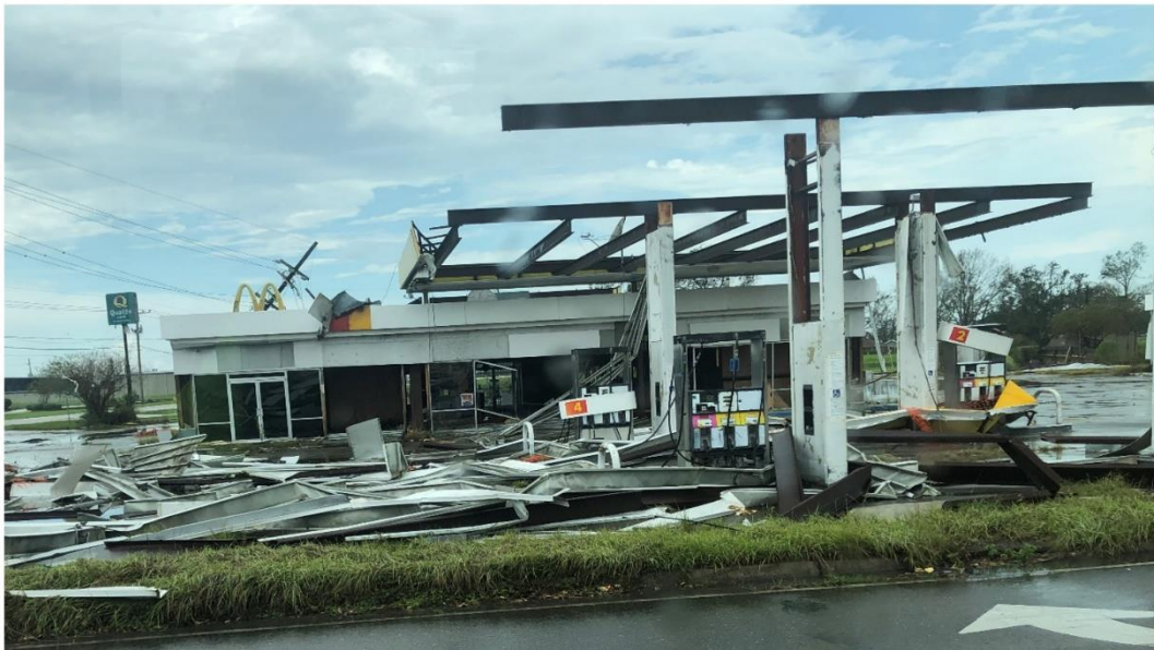
MI-TF1 performed wide area search operations, along with providing real-time Primary Damage Assessment for structures and identified critical infrastructure for local and state Emergency Managers during its deployment to Hurricane Ida.
